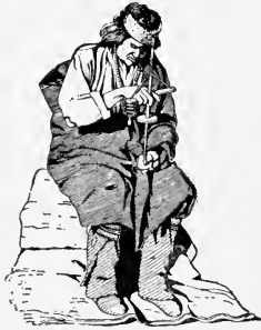
USE OF PUMP DRILL BY A ZUÑI
